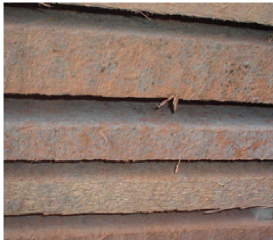
Figure 3: Mould on the Cocos nucifera drying timber
